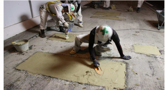
Patching by Repair Concrete
