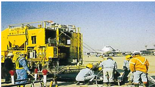
Repairing for apron of Airport
