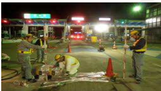
Repairing for Tollgate of Highway
