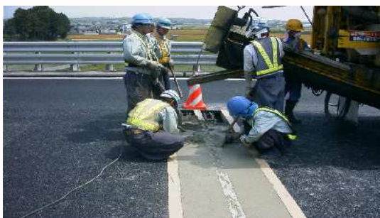
Repairing for expansion joint of Bridge
