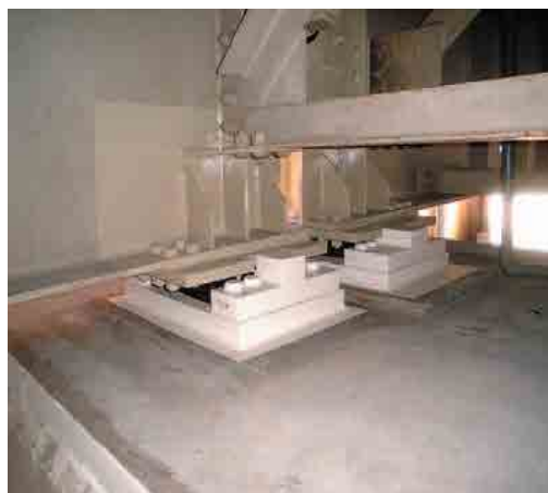
Grouting the base of heavy machinery with Pretascon
