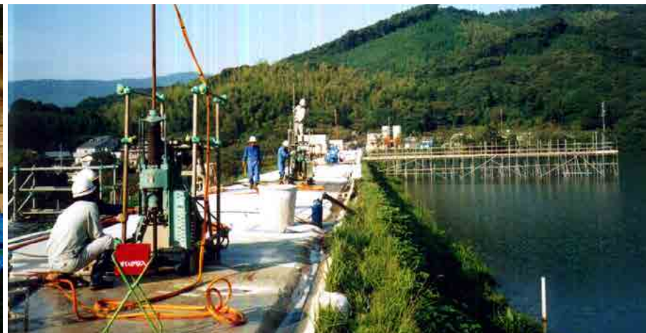
ES injection to ground for reservoir repair
