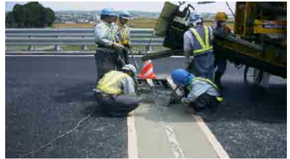
Repairing for expansion joint of bridge
