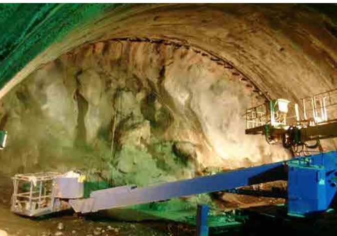
ES injection to the tunnel face
