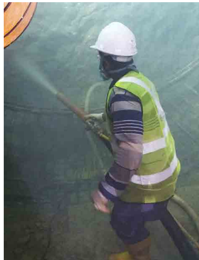
Spraying Subshot Mortar
