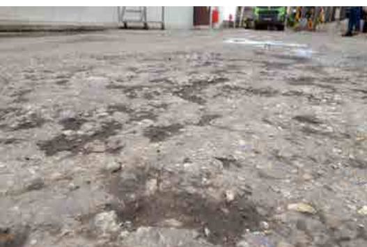
Existing uneven floor
