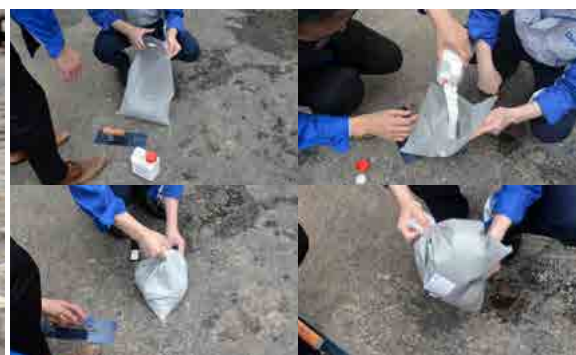
Mixing of Estopatch RSR
