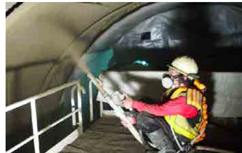
PF Mortar spray system in use
