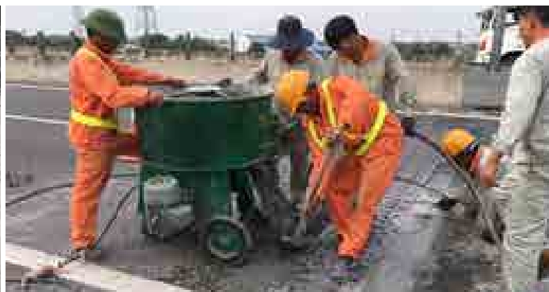
Mixing at site
